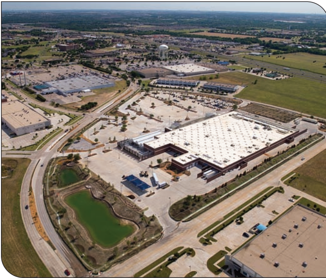
Walmart's experimental green store in McKinney, Texas features the latest in environmental, sustainable design including concrete parking lots and pervious paving.
