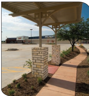
Sustainable Sites Credit 6.1. Light colored concrete panels
