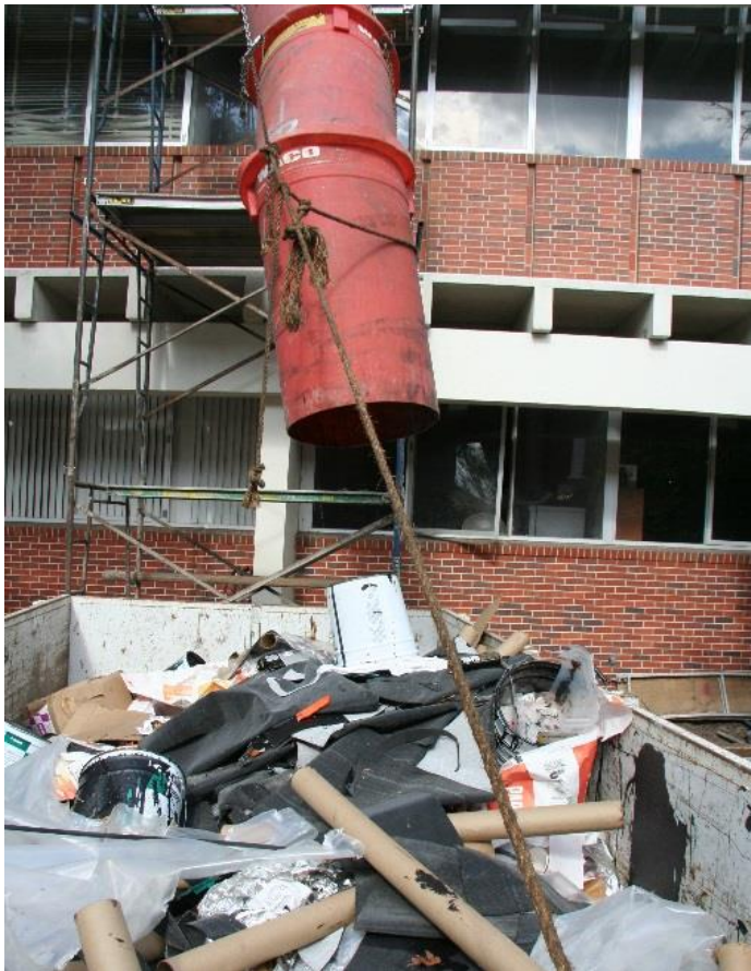
Figure 14. Building renovation with roll-off box and trash chute used to collect debris.
