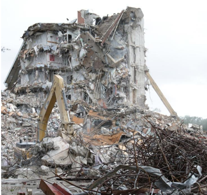
Figure 11. Building demolition with equipment collecting demolition debris.
