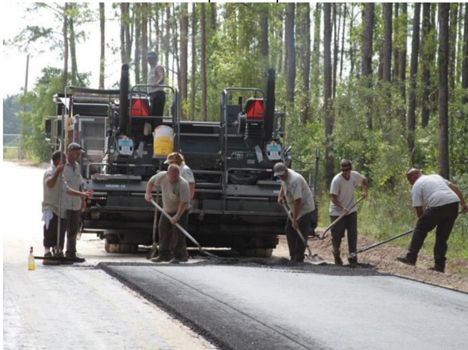
Figure 2. Asphalt concrete (or asphalt pavement) poured onto a road.
