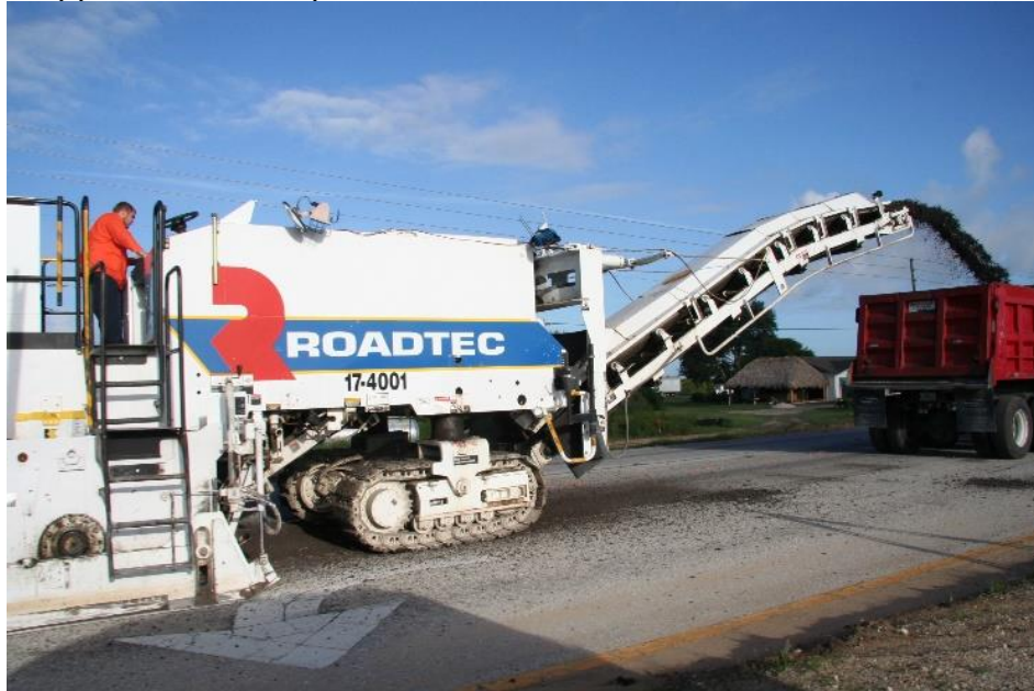
Figure 15. Reclaimed asphalt pavement collected and placed during road renovation.
