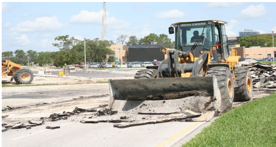
Figure 16. Reclaimed asphalt pavement collected during road renovation.
