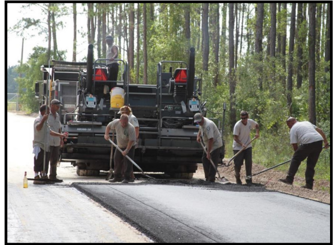
Asphalt shingles are commonly used in new asphalt pavement for roads
